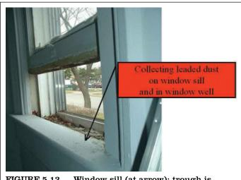
FIGURE 5.13 Window sill (at arrow); trough is behind sill, under sash and in front of storm window tracks. controls, maintenance or renovation. Some States, Indian Tribes, or local governments may require that window troughs be sampled as a part of a risk assessment.
