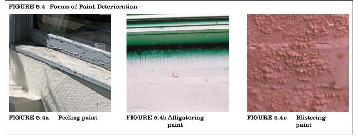
The following six types of paint deterioration are referred to as "layered deterioration."
