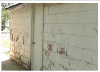
FIGURE 5.10 Soil lead hazard at dripline of garage.
